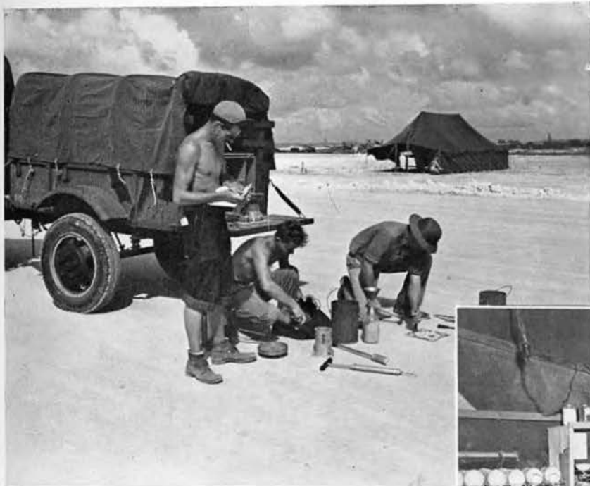
TAKING TEST SAMPLES OF NEW AIRSTRIP
