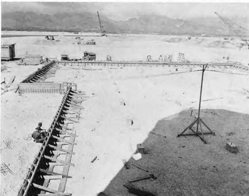
FOUNDATIONS FOR OPERATIONS BUILDING
