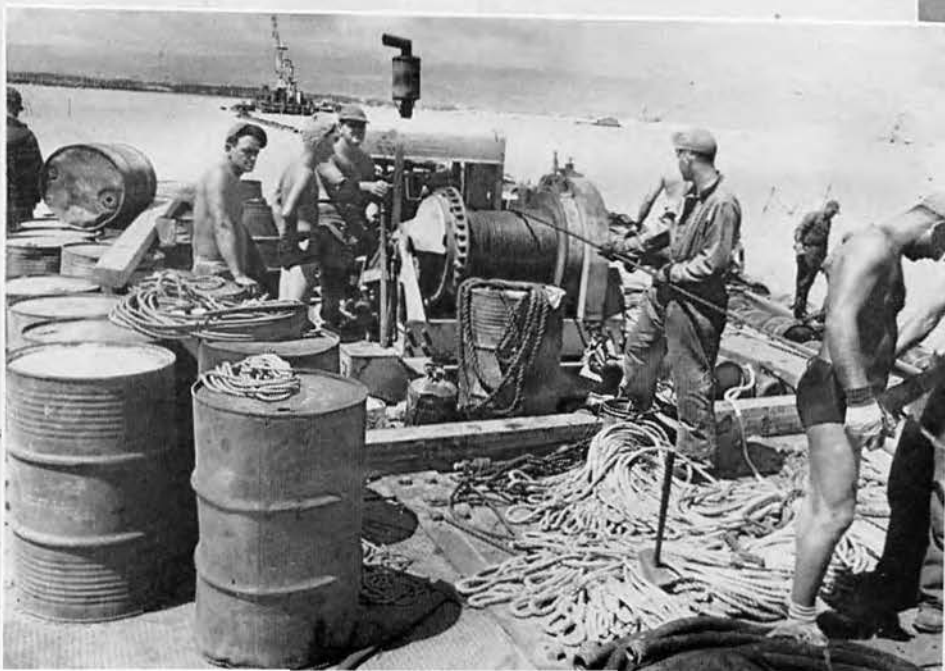
OPERATIONS ON MARINE OUTFALL SEWER
